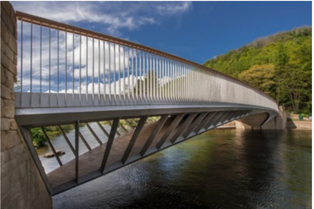
The 128ft replacement Pooley Bridge in Cumbria is the UK's first stainless steel single span bridge and was designed to avoid the need for piers in the river, making the structure more flood resilient. Photograph by Mike Smith
