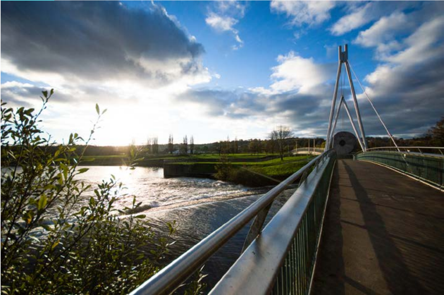
Blackaller Weir, Exeter
