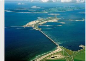
The Eastern Scheldt storm surge barrier was such an exceptional project that a new approach had to be taken to every part of its construction. A consortium of Dutch contractors was formed (Dosbouw) and cutting-edge methods and materials were used. Most of the prefabricated and construction works (piers, foundation mattress, storage of armour stone...) were carried out in the Neeltje Jans and a temporary bridge was built to connect the island to shore.
