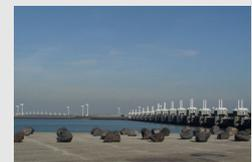
At the final stage, the service ducts, pier capping units, sluice-gates, sill beam and upper beam had to be put in place. The hollow service ducts, which would later be covered by a road, were laid on top of the piers. The ducts contain the operating and control equipment for the gates. The steel gates (from 6 to 12m high) were suspended between piers. The biggest sluice-gate weighs 480t. A specific barge-crane, the Taklift 4 was used for the installation of the gates.
