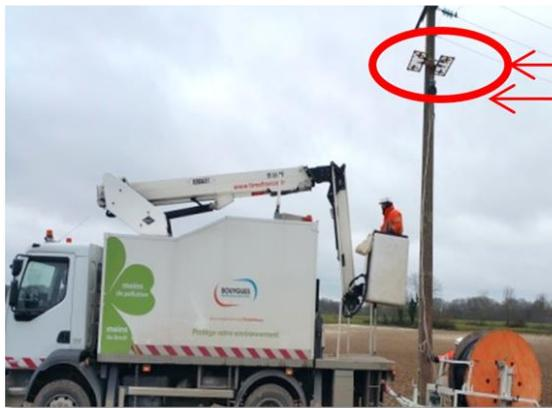
Shield to allow working on electrical pole , 'voltage on' (Internal Patent)
