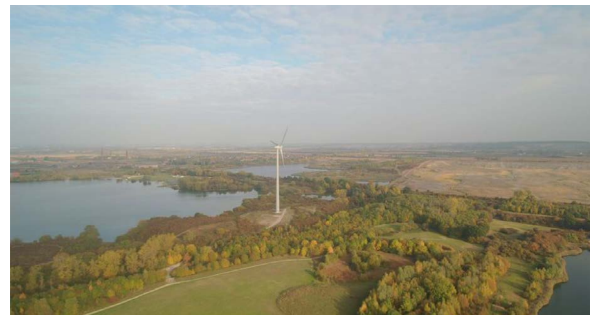
Aerial of forest of Marston Vale Solar PV Farm
